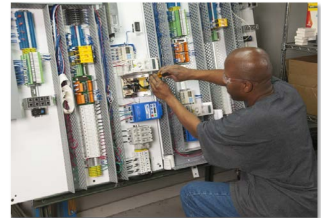
In-House Panel Build
